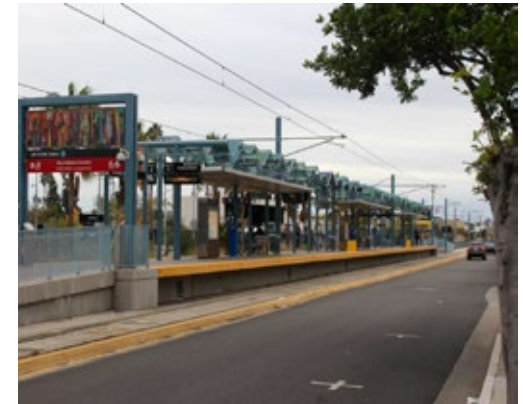
17TH STREET EXPO LINE STATION
