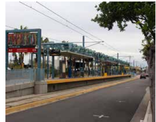
17TH STREET EXPO LINE STATION
