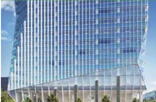
37 story office tower 700,000 SF office with supporting retail
